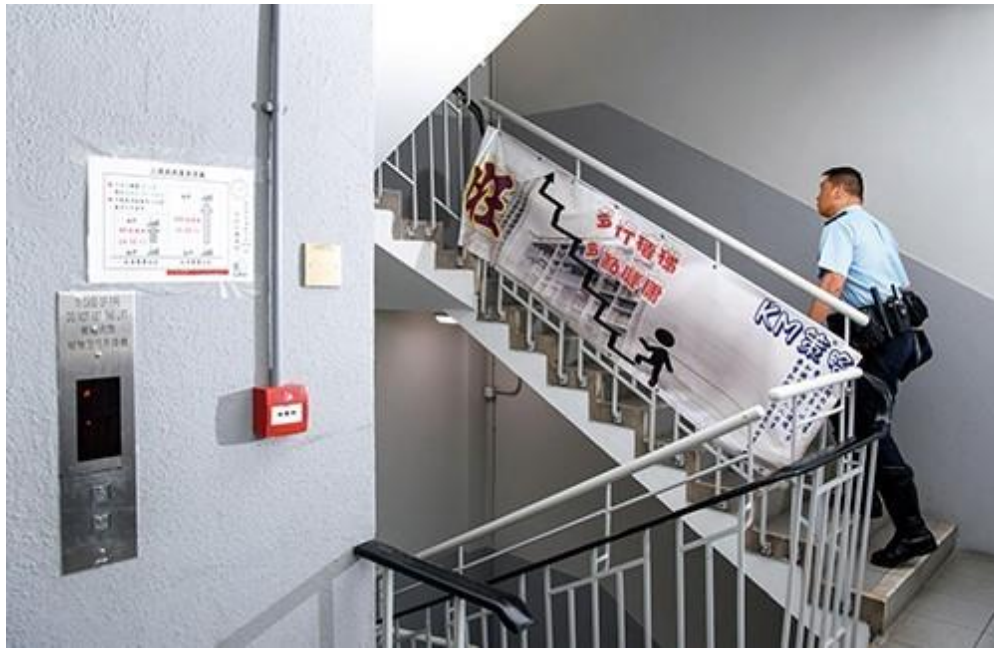
Banners are displayed to encourage staff to reduce their use of lifts and save energy.
