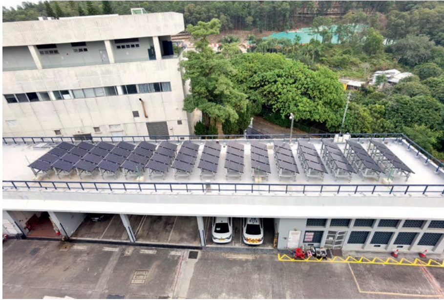
The Border District Headquarters harvest solar energy above its car park using photovoltaic panels.
