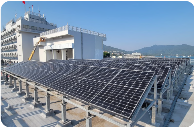
水警东分区基地和水警北分区基地的天台均装设光伏板。 PV panels harness solar energy on the rooftops of the Marine East Division Base and the Marine North Division Base.
