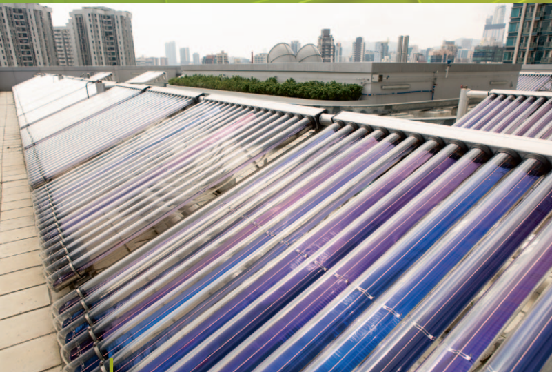
油麻地分区警署天台装设太阳能电池板，用作加热水温。 Solar panels have been installed on the roof of the Yau Ma Tei Divisional Police Station for water heating.
