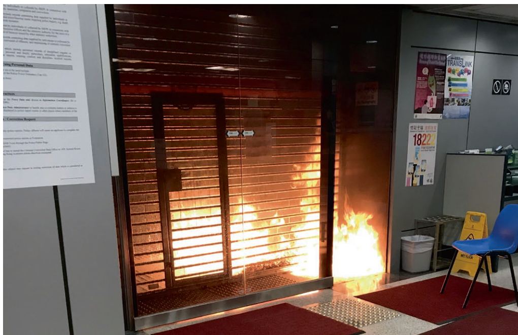
東涌警署報案室被投擲汽油彈，火光熊熊。 A fire caused by a petrol bomb attack on the Tung Chung Police Station Report Room.
