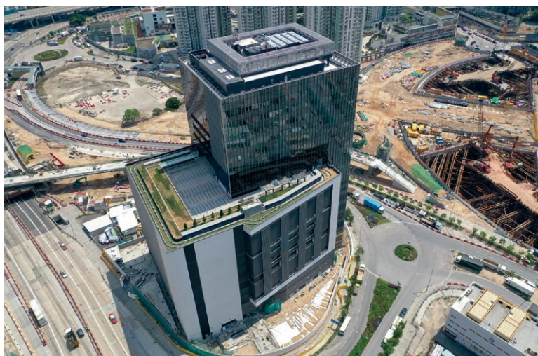
東九龍總區總部及行動基地暨牛頭角分區警署新貌。 A view of the Kowloon East Regional Headquarters and Operational Base cum Ngau Tau Kok Divisional Police Station.
