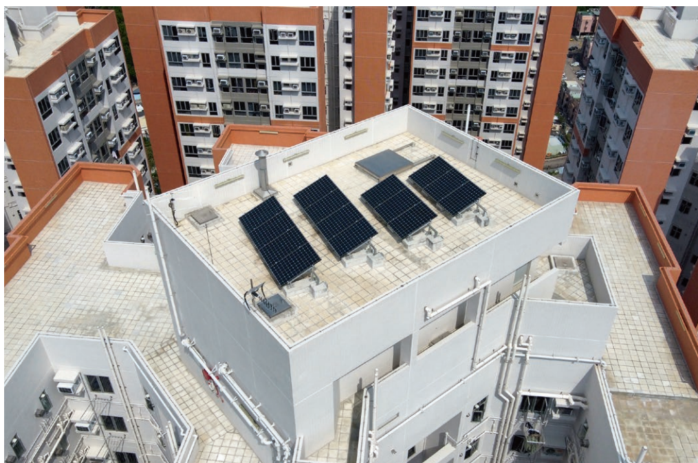
裝設於芬園天台的太陽能發電光伏板。 Photovoltaic panels are installed on the roof of a residential block at Fan Garden to convert solar energy to electricity.
