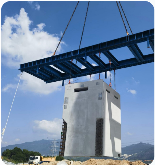
香港警察学院综合训练中心（缸瓦甫）的建筑工程涉及装嵌预制组件。 Construction of the Hong Kong Police College Integrated Training Centre (Kong Nga Po) involves installing prefabricated modules.
